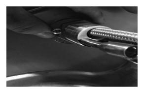
**Step six** – Feed Water Lines Though Lock Down Nut (L) and Hand tighten to counter.
