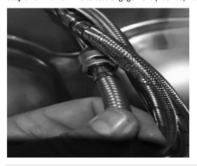
**Step three** – Attach Hot (red) and Cold (blue) supply lines hand thread the supply line and gently tighted with a wrench.
