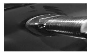
Step eight – Hand thread water lines to supply and gently tighten with wrench (Teflon tape may be used)
