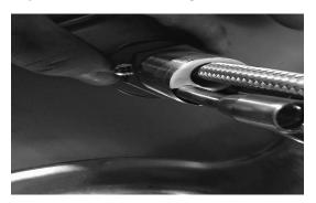
**Step seven** – Using Philips Head Screw Driver, tighten screws located on Lock Down Nut
